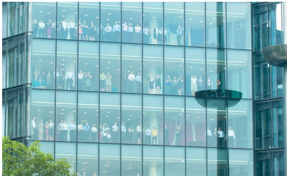
Offices in London Bridge
