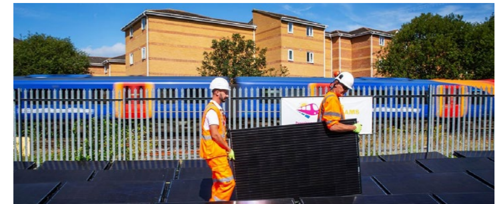
Installation of Solar Panels by Network Rail
