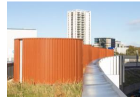
The Kings Cross Energy Centre
